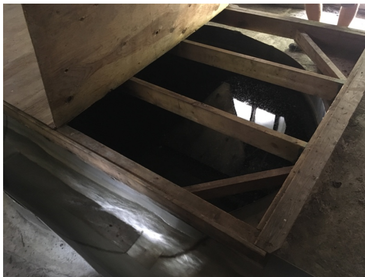
Figure 2 – Existing Reservoir Tank (1 of 2)
